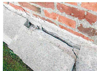
View of Sloped Top Concrete Facing
