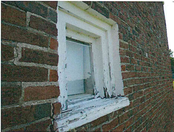
View of Existing Window to be Replaced
