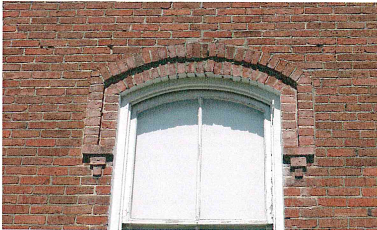
Projecting brick arched and dropped jambs
