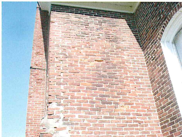
View of Brick Infill at Former Opening
