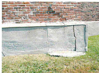
View of Concrete Facing
